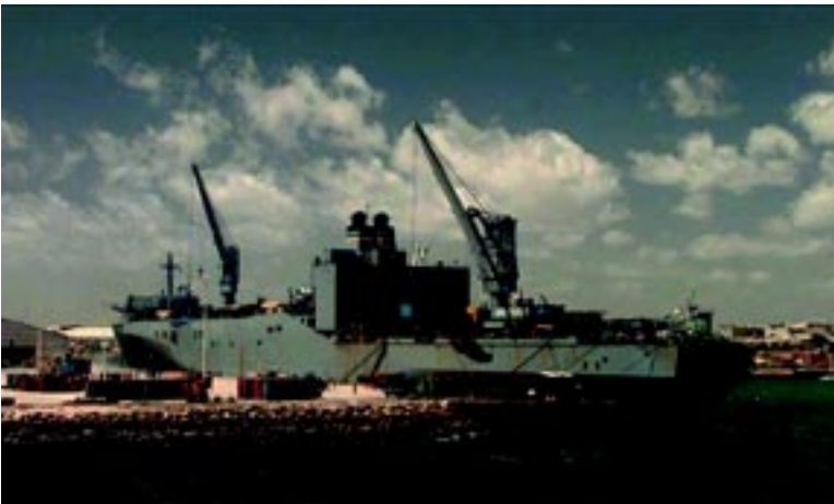
Surface lift provides up to 85 percent of the total dry cargo transportation requirements (90 percent if petroleum, oils, and lubricants is included).
